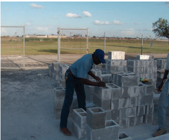
Myrick demonstrates the fundamentals of masonry.
