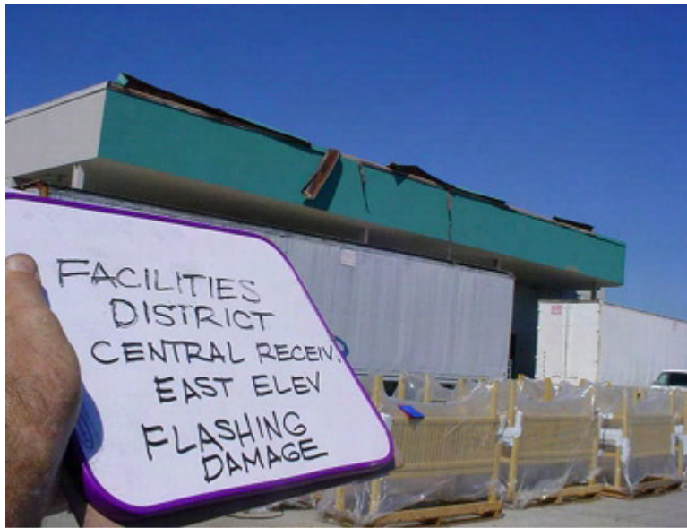
Photo 4 Photo Documenting Roof Flashing Damage
