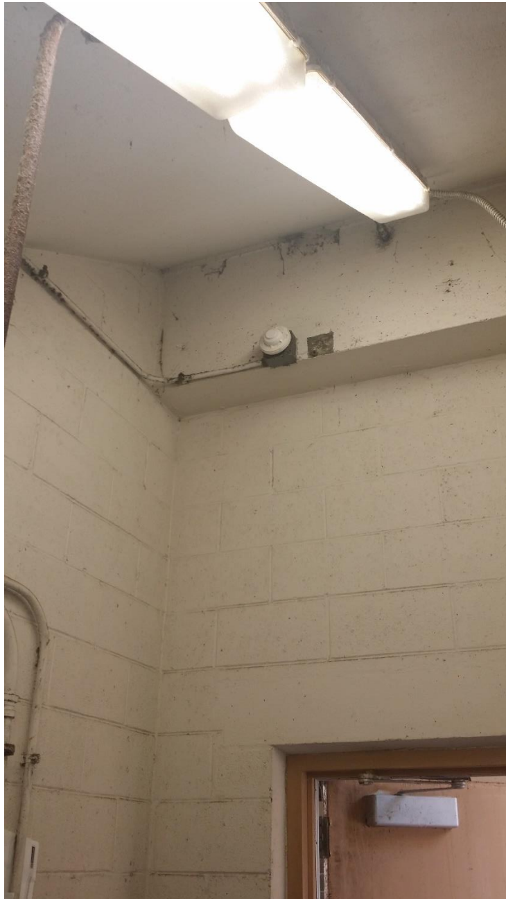
Existing smoke detector over machine room door.
