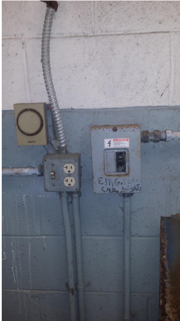
Existing 115vac outlet and switch in machine room Existing fan control
